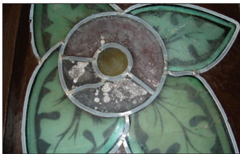
Fig.2. The XIV-th c. stained glass window with white organic deposit
