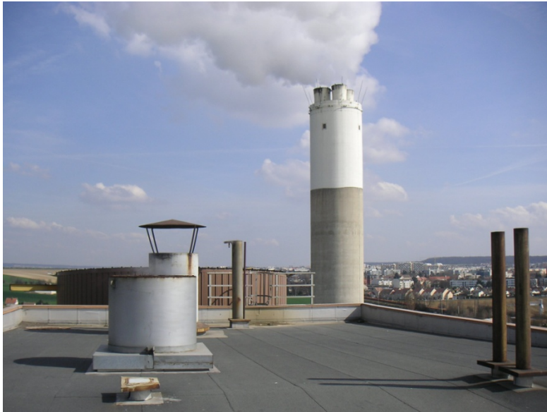
Stack seen from the roof
